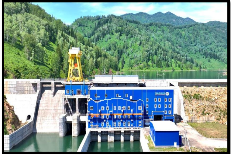
Turgusun hydropower station
